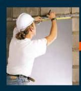
1 Measure the distance between the walls (brick to brick) and select the appropriate arch size. If renovating, remove existing plaster down to the masonry. Mark the centre of the aperture.
