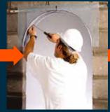
3 Fix the other sections in the same way, aligning them at the centre with the plastic joining pieces provided.
